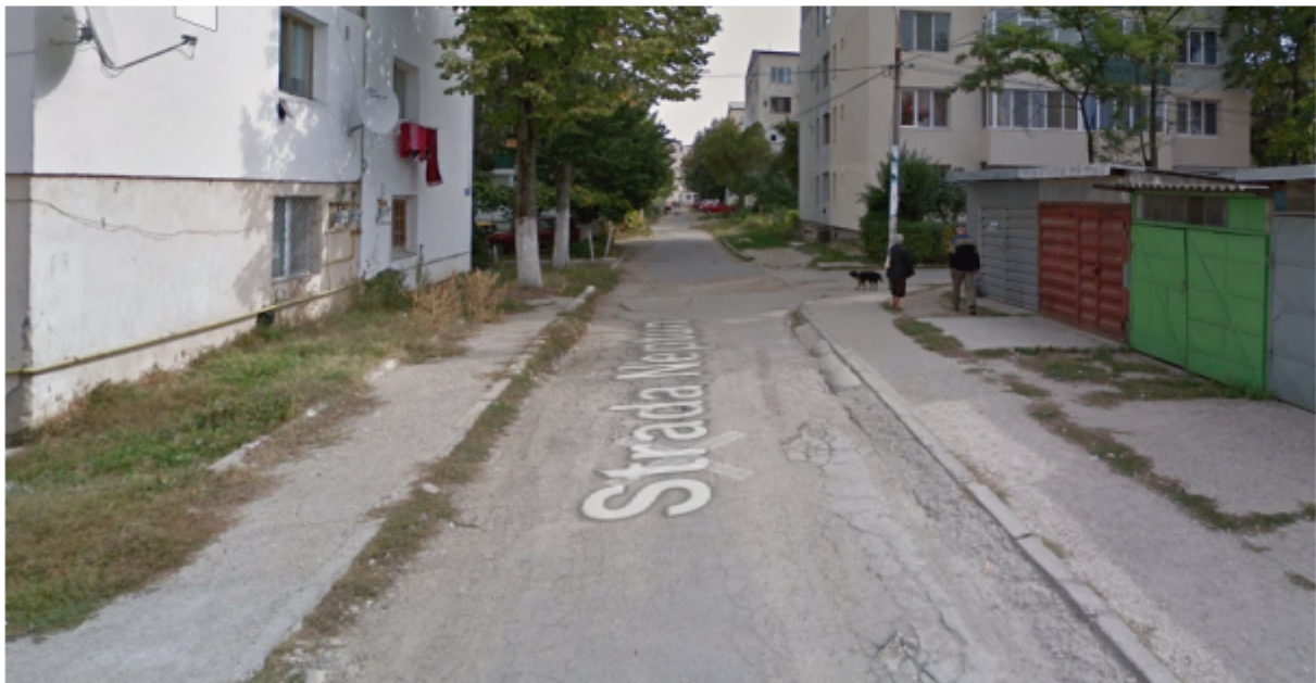
Drum nemodernizat, in partea sudica a zonei studiate.
