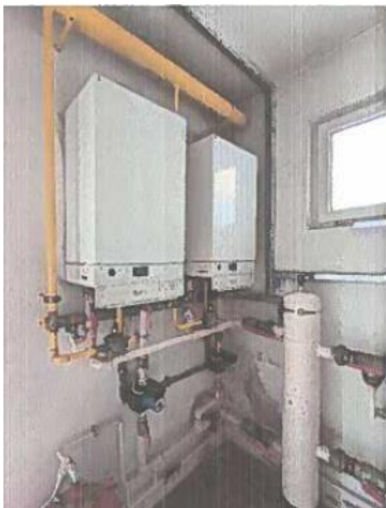
Photo 6 – Photo of the thermal system, one can see the two boilers providing heating and the boiler for storing the hot running water
