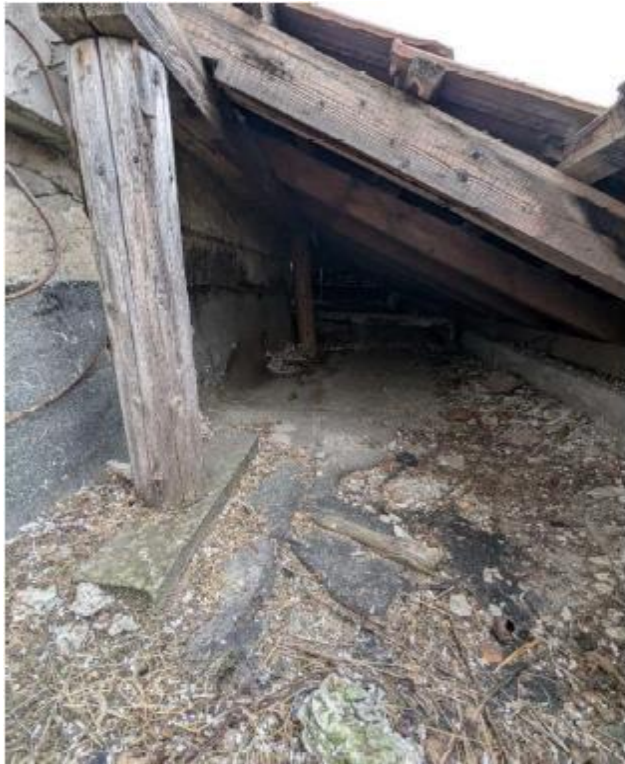
Photo 12 & 13 – The wooden truss over the groundfloor shows degradations, not being waterproof against rain
