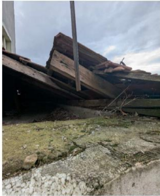
Photo 12 & 13 – The wooden truss over the groundfloor shows degradations, not being waterproof against rain
